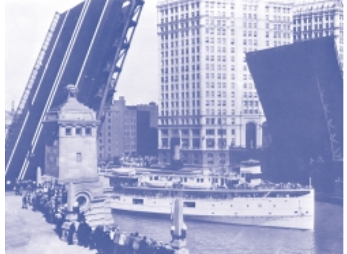
Bridge raising over the Chicago River
